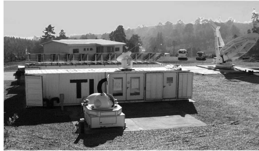
Figure 8.7. TIGO with SLR module (Concepción, Chile); courtesy BKG
