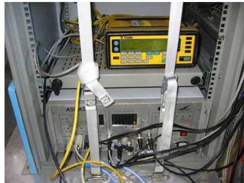
(b) ASIRAS instrument installed in the rack with AIR4 (Trimble 4000).
