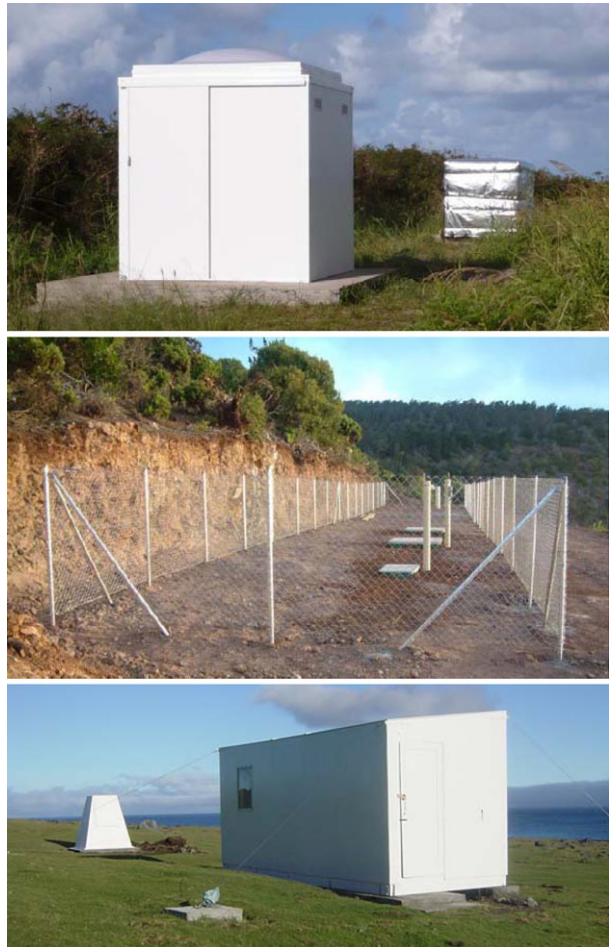
Fig. 8 Geomagnetic observatories on remote islands: Top : Easter Island with absolute hut in the front and variometer hut in the back (by courtesy of IPGP); Centre : St. Helena where the variometer and electronics are buried (by courtesy of GFZ); Bottom : Tristan da Cunha, with absolute hut and pyramid-shaped variometer box (by courtesy of DTU Space)
