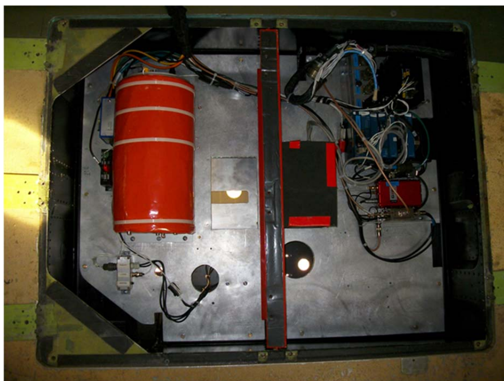
Figure 9: Instrument installation in the camera bay below the floor in the Twin Otter cabin; ALS (left), OXTS INS (middle right) and Trimble GPS receiver (lower right). Note ALS and OXTS INS axis are mounted along aircraft centre line. Installation: Forward to left. Aircraft right is at the top.
